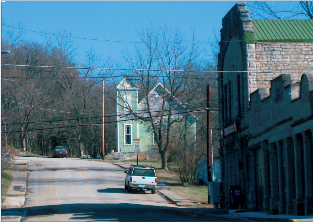
WITH THE AID OF A LOW-INTEREST LOAN FROM BLOOMINGTON RESTORATIONS, INC. (BRI), A LOCAL PRESERVATIONIST RESTORED THE QUEEN ANNE-STYLE CHURCH UP MAIN STREET FROM THE STINESVILLE MERCHANTILE.
